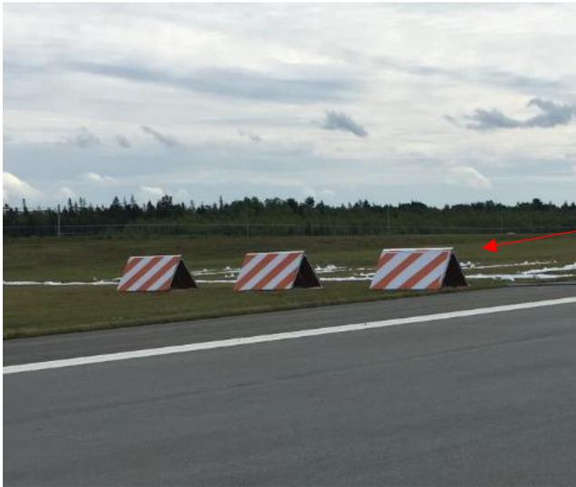
High barricades used to identify the threshold.
