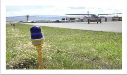
A photograph of a blue edge light mounted on a yellow post, situated on a grassy field. In the background, an airport terminal and aircraft are visible under a clear sky.           |
