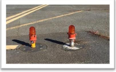
A photograph showing two amber lights mounted on a yellow base, positioned at the intersection of a taxiway and an apron. The lights are illuminated and cast shadows on the asphalt. |
