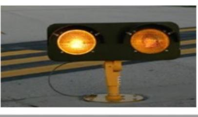
A close-up photograph of a runway guard light. It features two glowing amber lenses mounted on a yellow base, positioned at the intersection of a taxiway and a runway.             |
