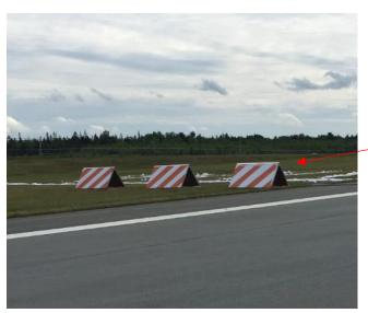
High barricades used to identify the threshold.
